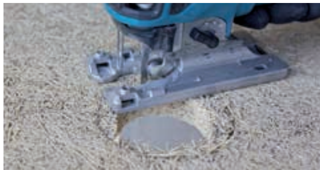
Cutting out an aperture with a jigsaw, tile face side down.
