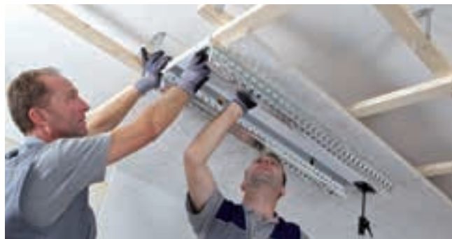
Alternative: Fix the ceiling light using screws into the wood battens or SD profiles at the sides or direct attachment into the ceiling.
