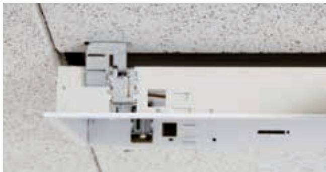
Hang the ceiling light. Fix with the supplied side wings to the T-profiles, CD profiles or wooden battens. Adjust the installation height of the light to the existing suspension height.
