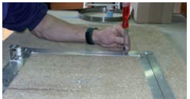
Fix the cover tile with min. 2 x 4 number screws 4.5 x 20 mm per frame 40 x 40 or 2 x 6 number for 60 x 40 cm and Heraklith-BM PU or polymer glue on the inner frame.
