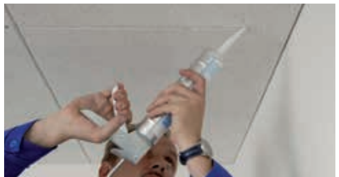
HERADESIGN® micro acoustic tile joints can be filled using Knauf acrylic sealer and can be painted over with silicate paint.
