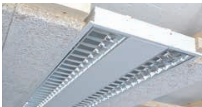
The joint between the Heradesign acoustic tile and the light is covered by the frame.
