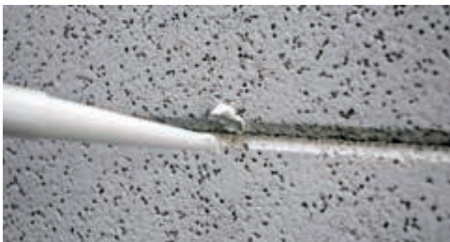
Touching-up small imperfections of HERADESIGN® micro or HERADESIGN® plano acoustic tiles: Fill the imperfection/chipped edge with acrylate or wood filler, scrape off the excess with a trowel and cover with the same paint as the tile when it's dry.
