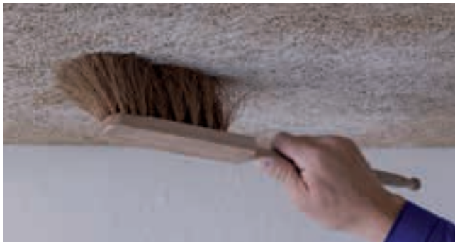
Brushing: Efflorescence, dust, etc. can be removed with a soft brush. Set loose fibres with StoPrim Plex primer.
