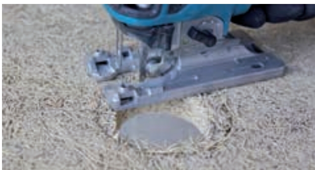
Jigsaw Lay the acoustic tile face side down. Always make cuts with a guide.
