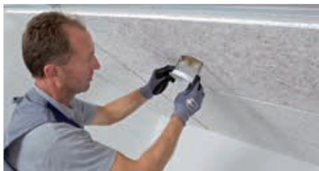
Insertion of the spotlight housing.
