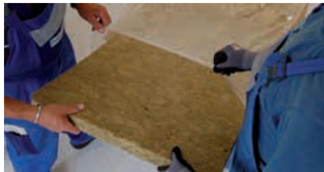
Slide in the acoustic overlay.
