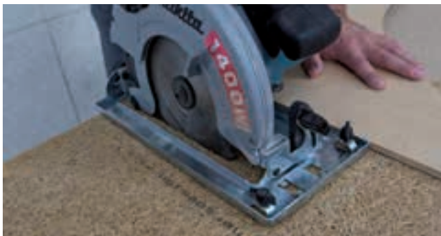
Circular saw Lay the acoustic tile down face side down. Always work with a guide and an extraction system. Support the free end of the tile.
