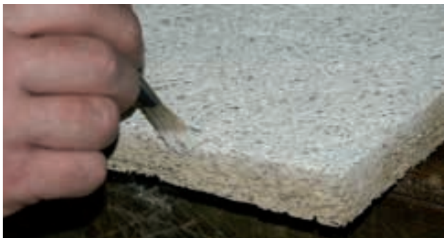
Paint the edges.
