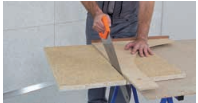
Jack saw Lay the acoustic tile down face side up. Always work with a guide. Support the free end of the tile.
