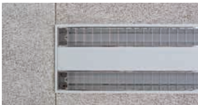
Installed modular light. The tile joint is covered by the frame.
